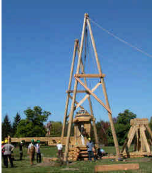
Twin A Frame lift to position 8.5 tonne catapult body on its stand
