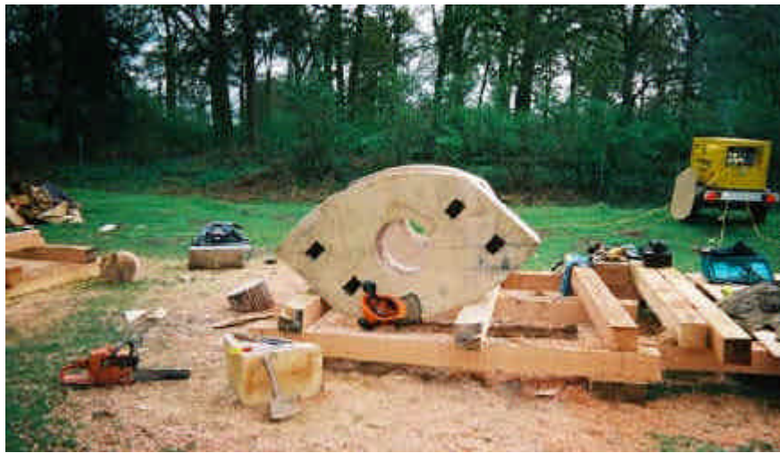
Torsion spring and arm assembly
