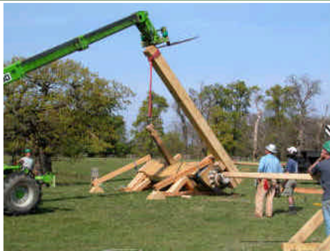
Pre-rotation of spring cassettes to wind in spring tension (up to 200 tonnes per spring)
