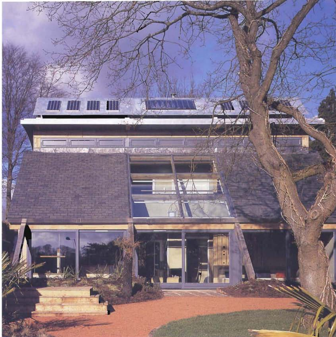
Above The south front is topped by solar water heating and photovoltaic panels.
