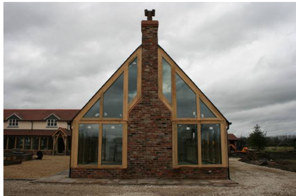
Fig 3: Unusually shaped units can more easily be accommodated when surface mounted
