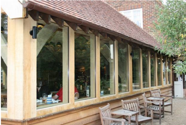
Fig 2: Surface mounted glazing; a series of fixed glazing panels mounted onto studs and then faced with an oak cover board. Note the visual effect is that the glass is recessed into a single stud.
