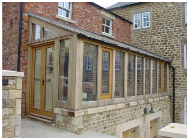
Fig 5: A small lean-to sunroom with joinery doors to the end gable, and two opening windows. Note the visual appearance of these and the surface mounted panels.
