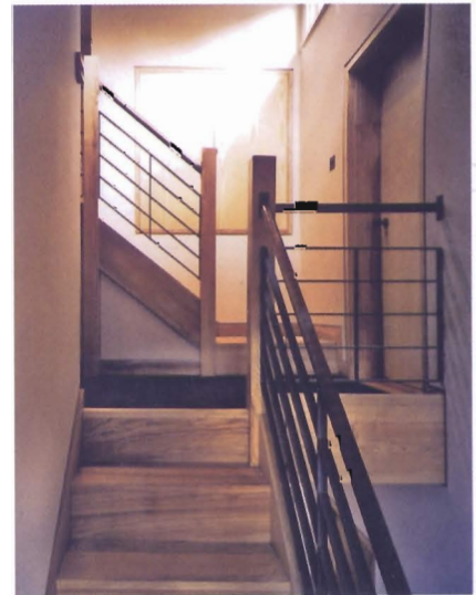
Figure 2.8 The ash staircase replaces one that had rotted
