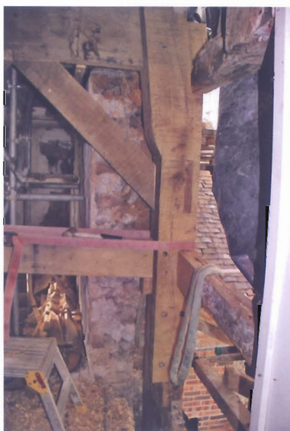
Figure 2.15 New for old Photo: Carpenter Oak & Woodland
