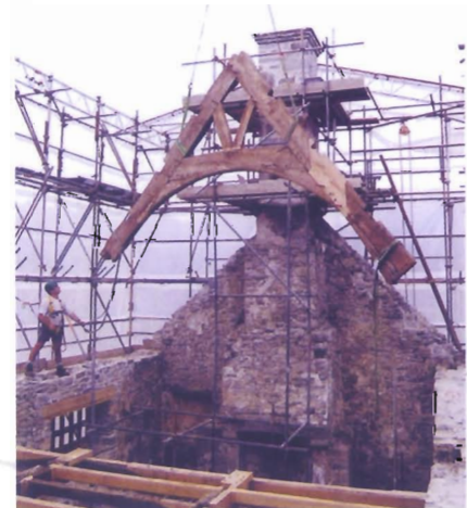
Figure 2.9 A restored truss is lowered into position at Dobelydr
